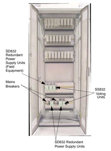
Figure 5.3: Floor Mounted Cabinet - Unit Arrangement (Redundant PSU)
