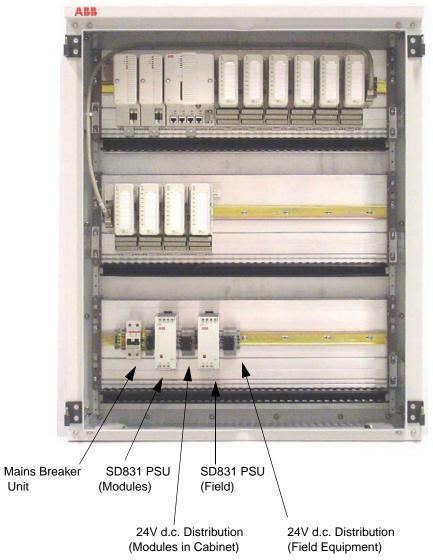
Figure 5.2: Wall Cabinet - Dual Power Supply (Local/Field) Arrangement
