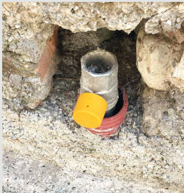
Something that would be unthinkable in Germany: A gas connection with no blind plug – discovered by Luciano Schrecke-Chiacchiararelli at Lake Garda in Italy.
